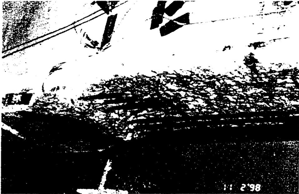
**Figure 4.76. Damaged Bottom Flange of Beam 2, Removed Strands in Foreground.**
